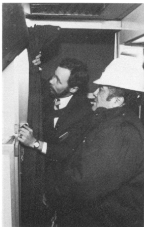
On a pre-trip inspection, Train Chief Paul M. Clements (left) and Mechanical General Foreman Louis Maldonado check a bed latch.
