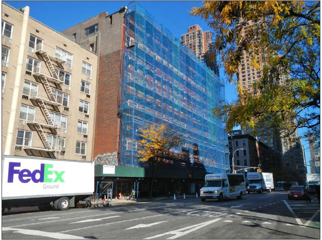
View northwest to the Windermere from Ninth Avenue 3
