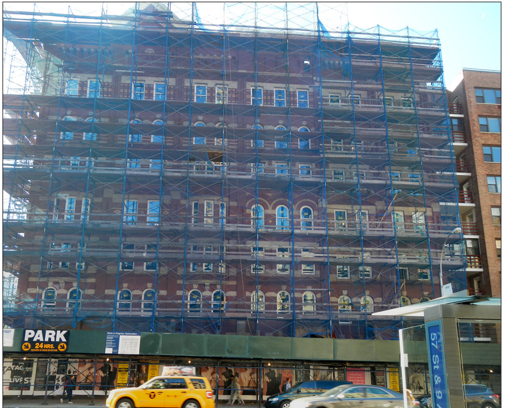
View south on West 57th Street to the Windermere's north facade 2
