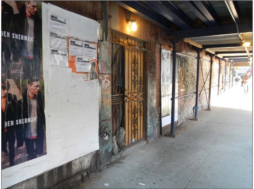
View to the Windermere's ground floor façade 4
