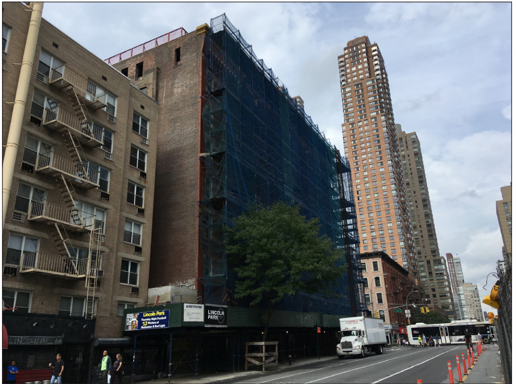
View northwest to the Windermere from Ninth Avenue 2
