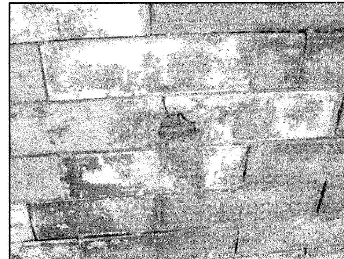
P3 TYPICAL ANCHOR TO BE REMOVED N.T.S.
