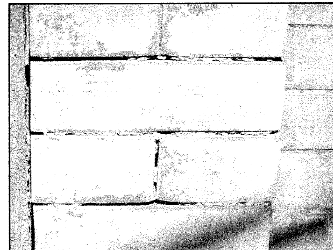
P2 TYPICAL OPEN MORTAR JOINT N.T.S.
