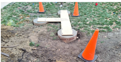
Three cylinders go 3-feet deep to hold the statue in place.
