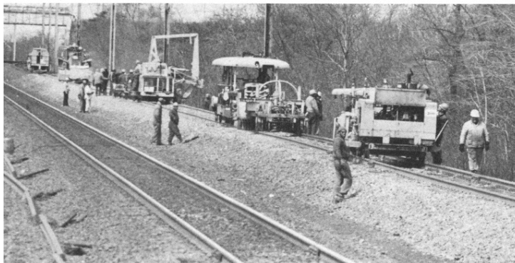
Track machinery, strung out in a long line in the Corridor, works on upgrading the track for future 120-mile-an-hour train speeds.
